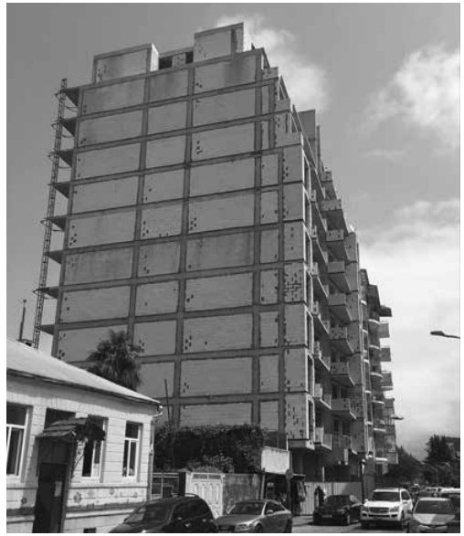
Fig.3 An incomplete twelve-storey building dwarfs its neighboring traditional Adjara-style single family home in Batumi's Old City.
